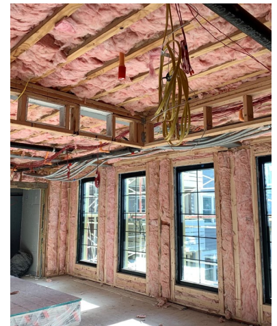
Insulating Co-Working Space in Building A
