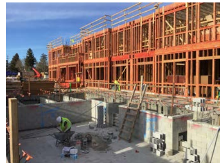
Pool foundations and framing work
