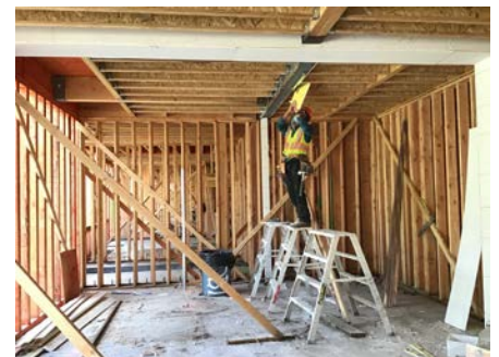
Construction in progress
