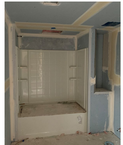
Shower Installation in Building A
