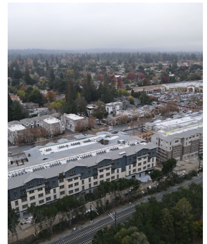
Aerial View of Construction Site
