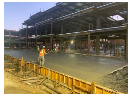
Office Building 2 Foundations Concrete Pour
