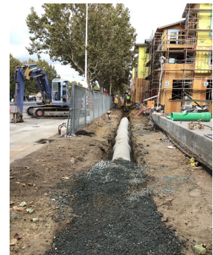
Storm Drain Installation
