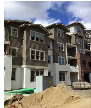
Touching Up Building B Exterior
