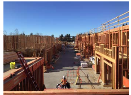
Upper level framing in progress
