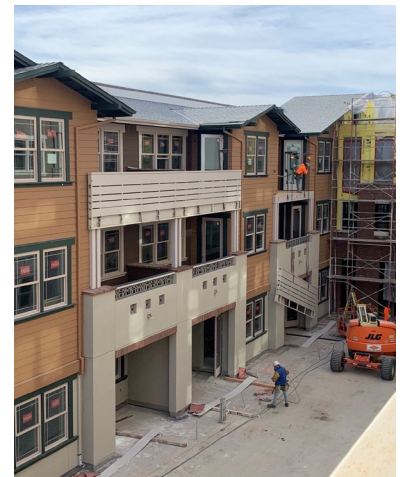
Balcony Railing Work Continues at Residential Building A
