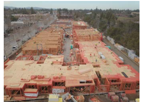
Aerial view of construction site
